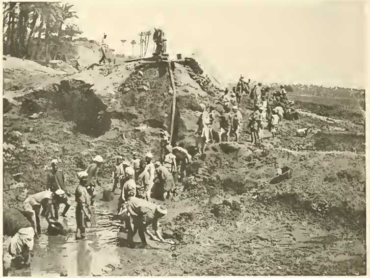
PUMPING OUT THE POND.
